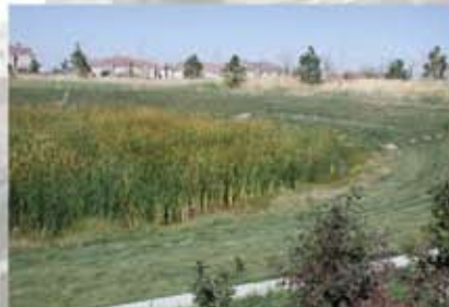
Stormwater Detention Pond
